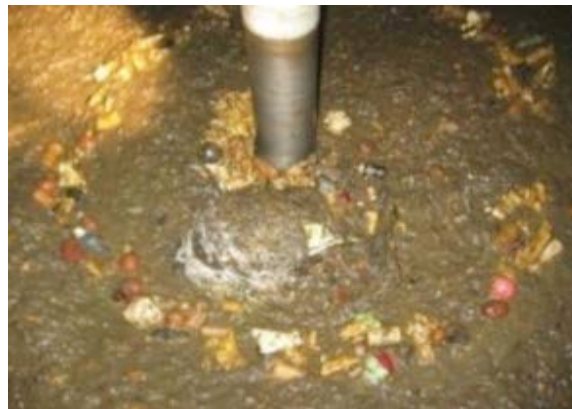
MIXING SLURRY PREPARATION
